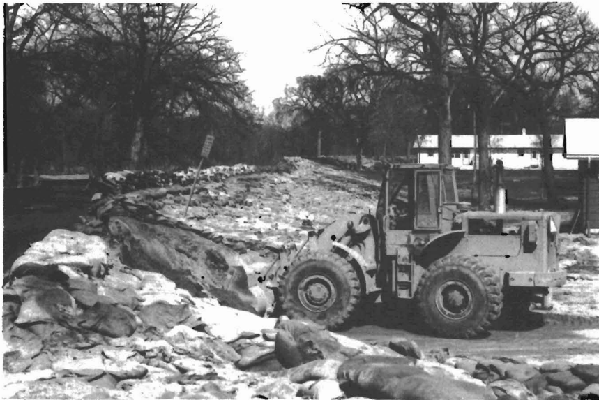
Figure 3. Riverside Park area showing dike cleanup. The cost of cleaning up after a flood is also considerable. Volunteer labor generally “dries up” as soon as the crest is reached. This dike is in the Riverside Park area.
