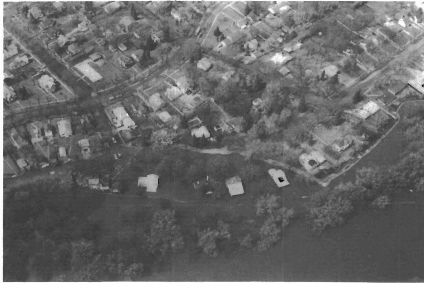
Figure 20. An air view of the Riverside Drive area during the 1979 flood. Four homes were heavily damaged there during the 1979 flood when a dike gave way. The expense of protecting these homes from nearly every flood has been a point of considerable controversy. Photo by Lee Clayton.
