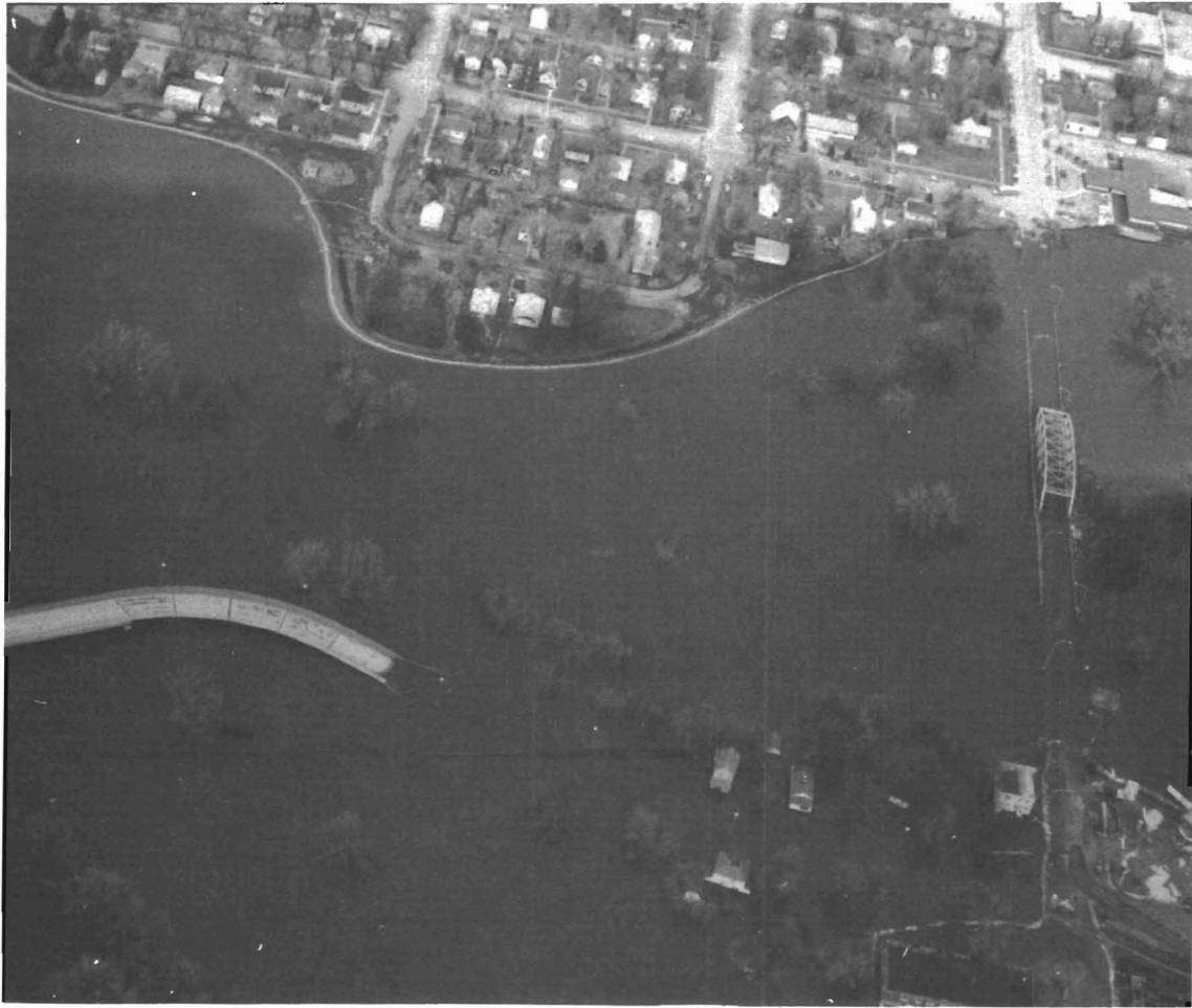
Figure 28. Minnesota Point, East Grand Forks. The end of the Minnesota Point Bridge and nearly all of the roadway of the Red Lake River Bridge were submerged during the April 1979 flood. The river level shown here is approximately 49 feet. Photo by Lee Clayton.
