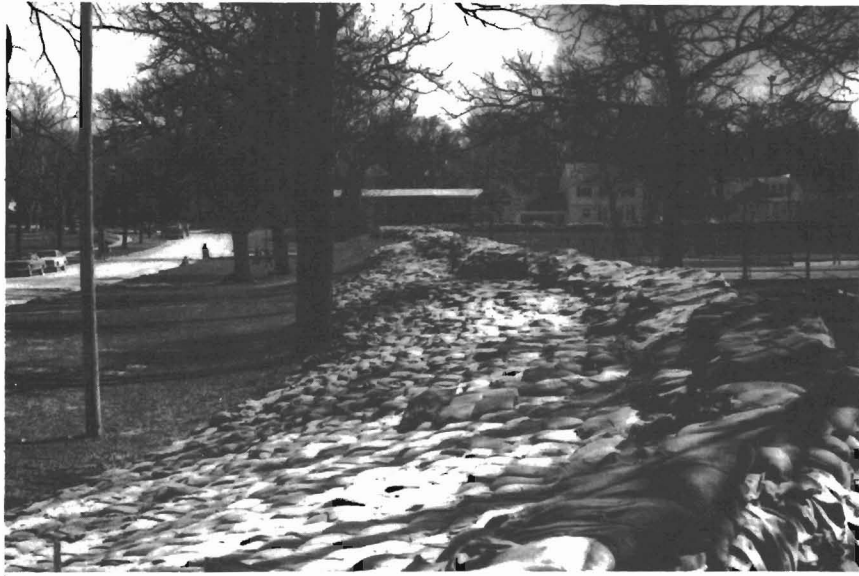
Figure 2. Riverside Park area showing sandbag dike. The expense of building massive sandbag dikes can be staggering. This dike (picture taken after the water receded) is near Riverside Pool, which was permanently closed as a result of damages sustained during the 1979 flood. Over 5 million sandbags were used in Grand Forks-East Grand Forks in fighting the 1979 flood.
