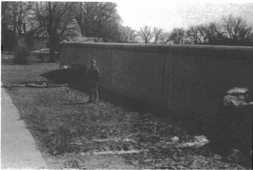
Figure 45. Two views of the south end of the Lincoln Park dike in Grand Forks during the 1979 flood. This dike includes 770 feet of concrete floodwall and 5,160 feet of earthen levee. It protects the Lincoln Drive area against a flood of 52 to 53 feet.
