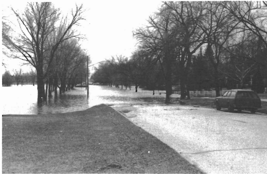
Figure 18. Belmont Road at the 1300 Block. View south, during the 1979 flood.
