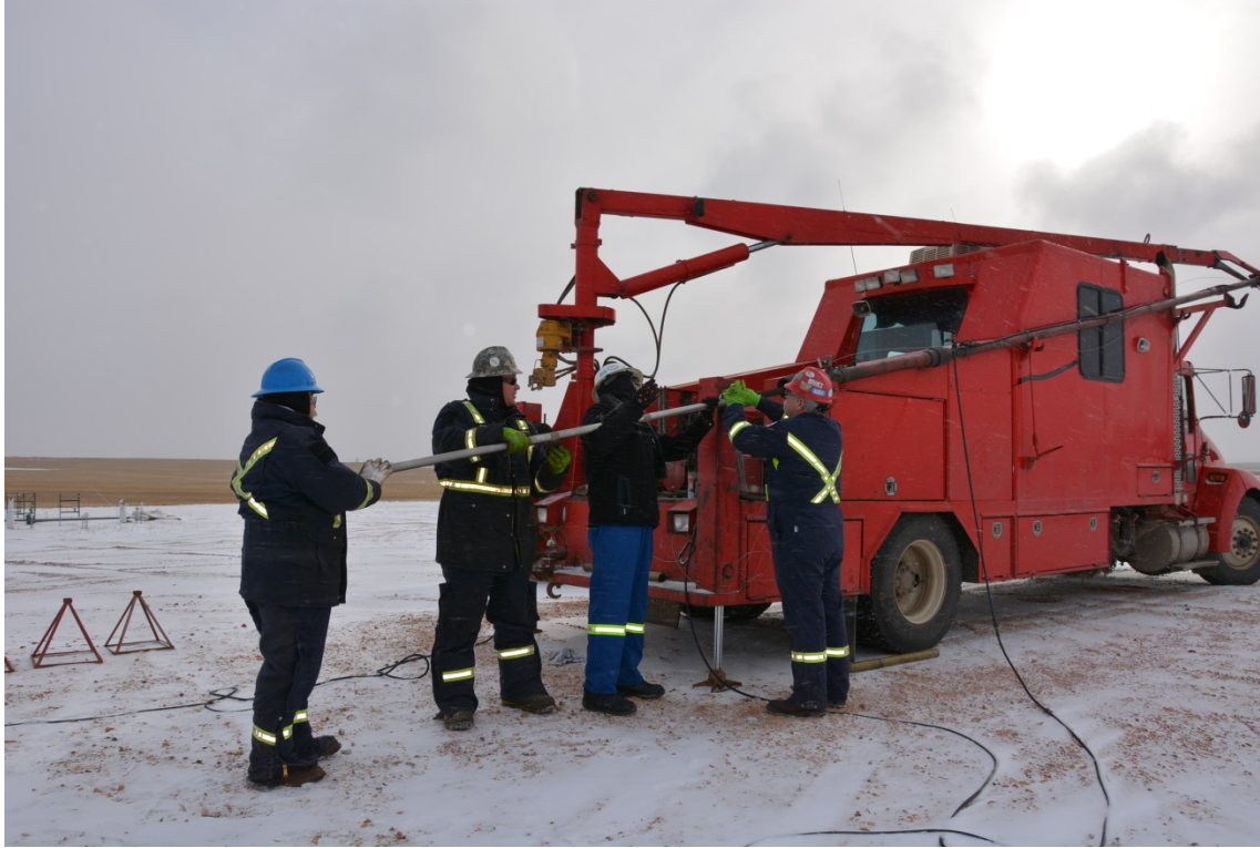
Figure 2. Connecting the tool to the slickline. From left to right: Mike Harden, WISCO, David Smith, WISCO, Jay Jamali, GOWell, and Kevin Hammer, WISCO.
