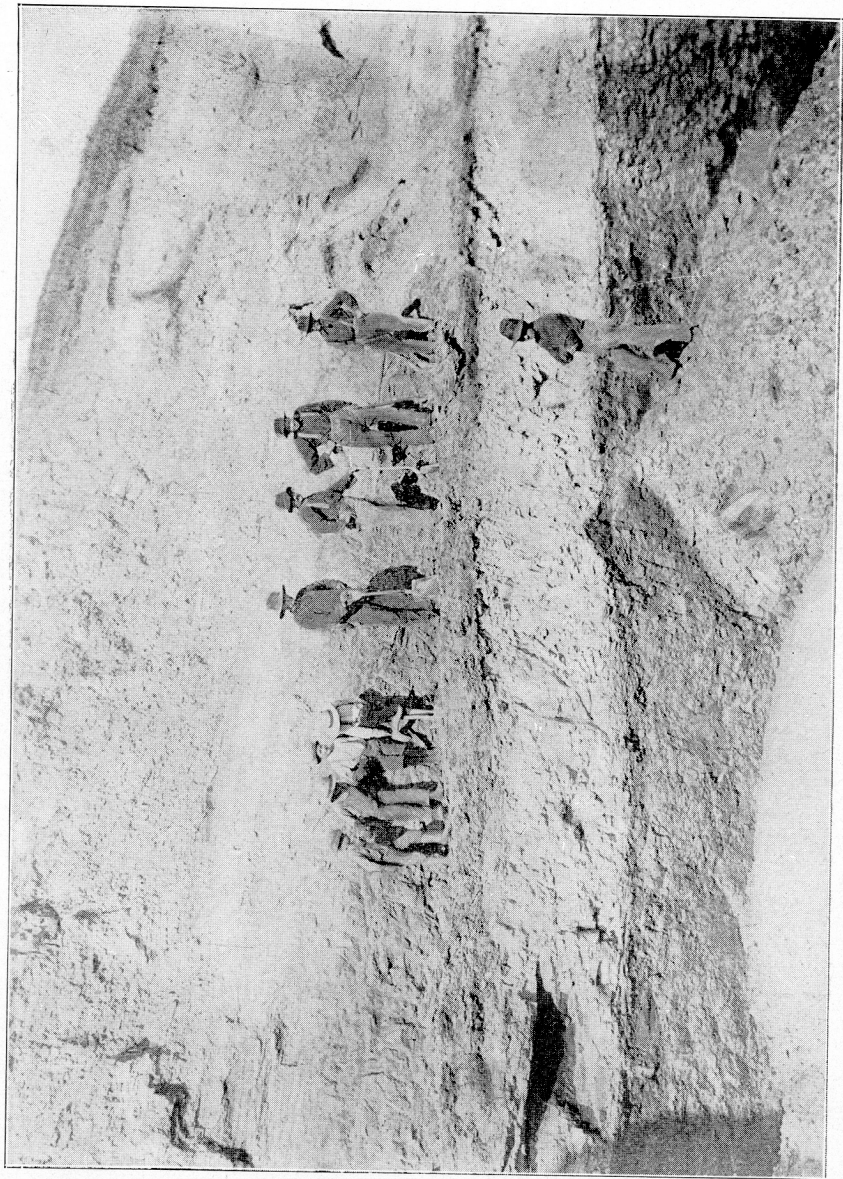
Lignite in the Pit of the Dickinson Fire Brick Company. The Upper Clay Is Used for Brick While the Lignite is Used for Fuel in the Kilns.
