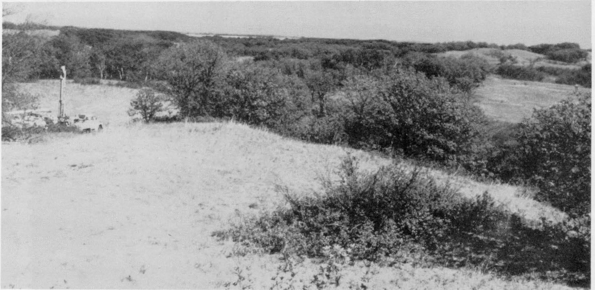
Figure 11. Augering testhole for monitoring well 6. View is to the southeast.
