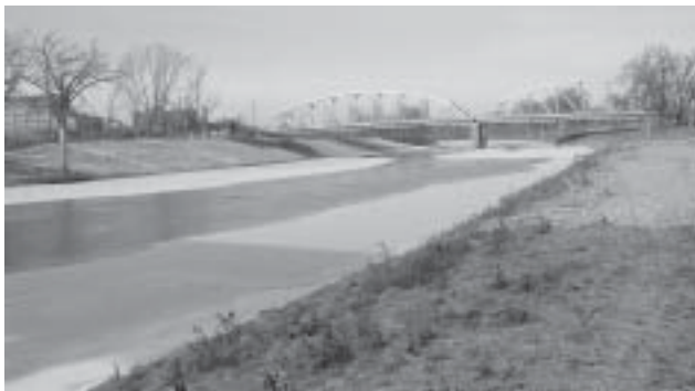
Figure 2. North Dakota - Minnesota boundary. Sorlie Bridge across the Red River of the North at Grand Forks, ND - East Grand Forks, MN. The view is downstream, with Grand Forks, North Dakota on the left. The Sorlie Bridge was named for North Dakota Governor Arthur Sorlie of Grand Forks and dedicated in 1929. Photo by John Bluemle.
